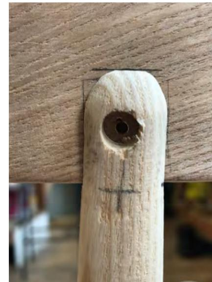
Back joining holes marking
