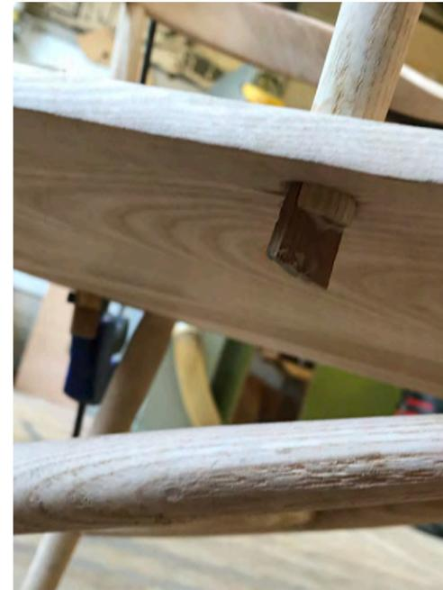
Spindles wedge jointed & glued
