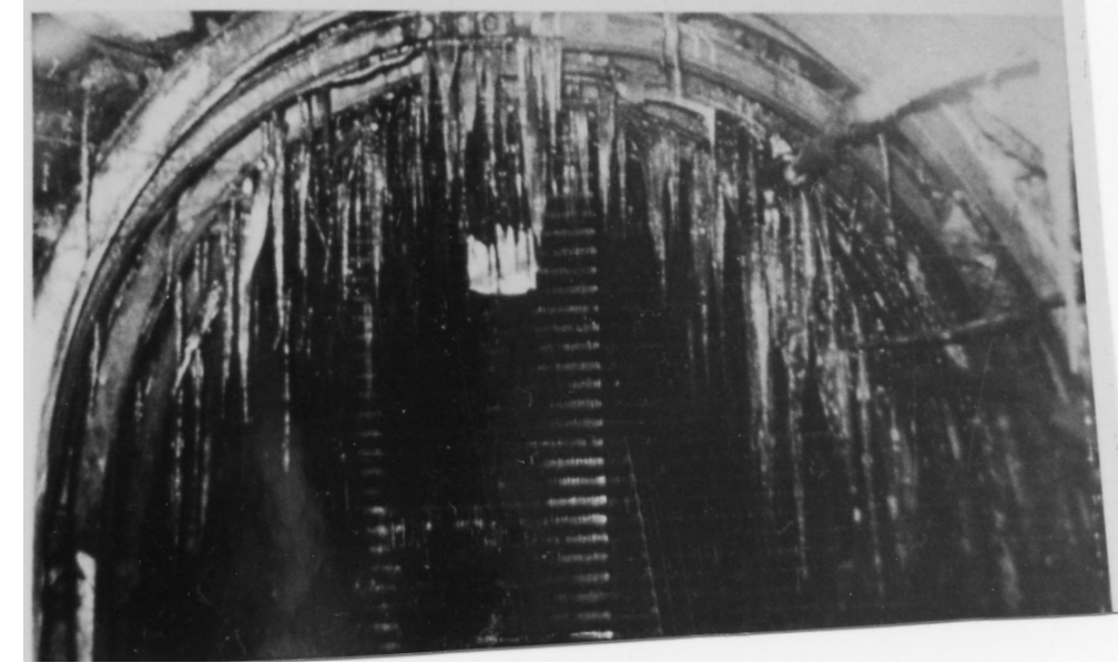
Photo taken by my great Grandad of the inside of a mine he was working at in Port Talbot. The square patch of light in the middle is the door way out and the long shards hanging from the ceiling are icicles.
