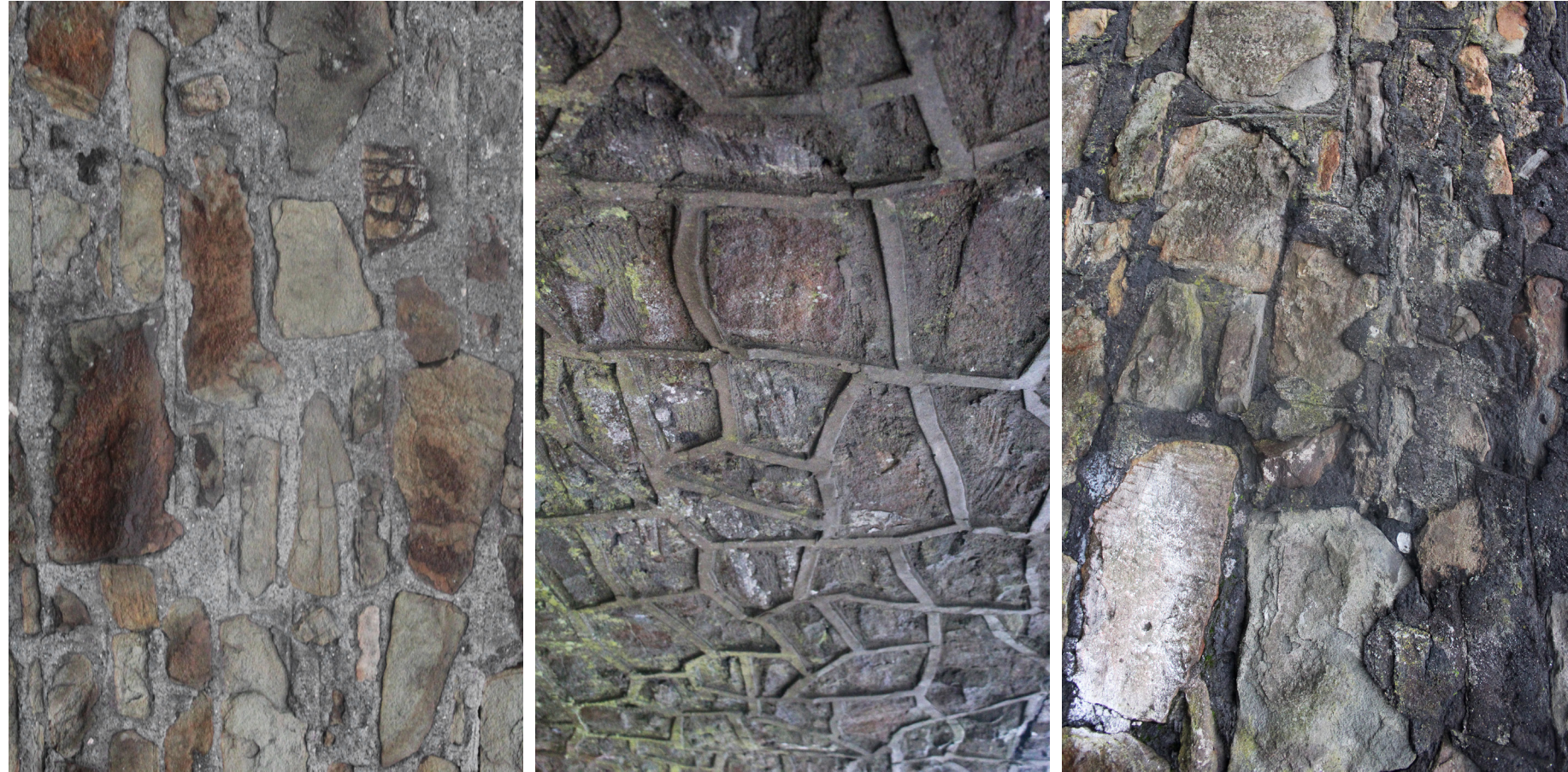
Photographs taken of stone walls and buildings close up around Port Talbot's town.
