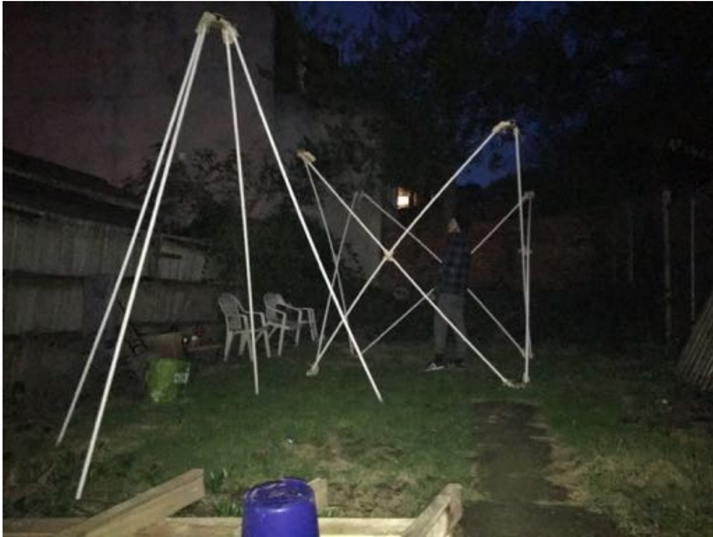
Test Build with 3m PVC pipes. The pipes were too flexible over a 3 meter length to complete the structure, but it was a successful build whilst the hubs worked successfully to hold the structure together.
