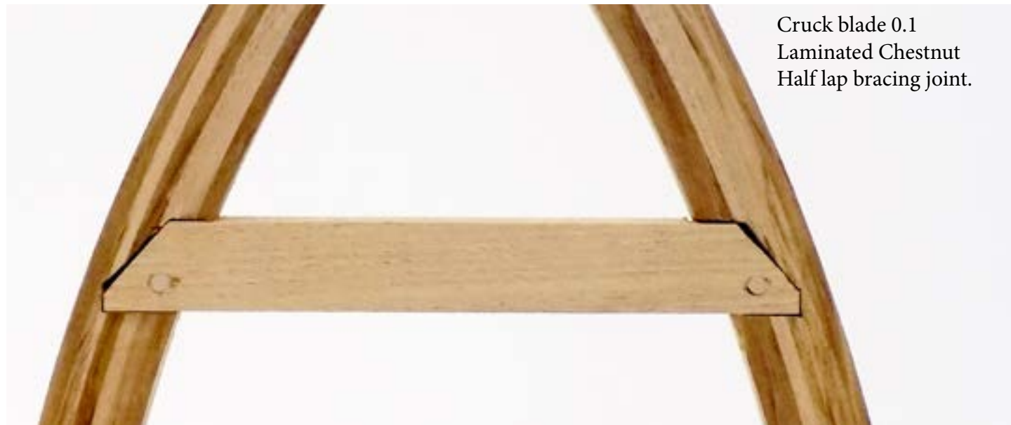
Through peg joint Exposed
