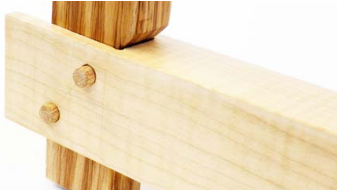
Cruck blade 0.1 Laminated Chestnut Half lap bracing joint.
